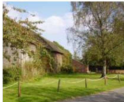
Overton Hall Farm Barn
